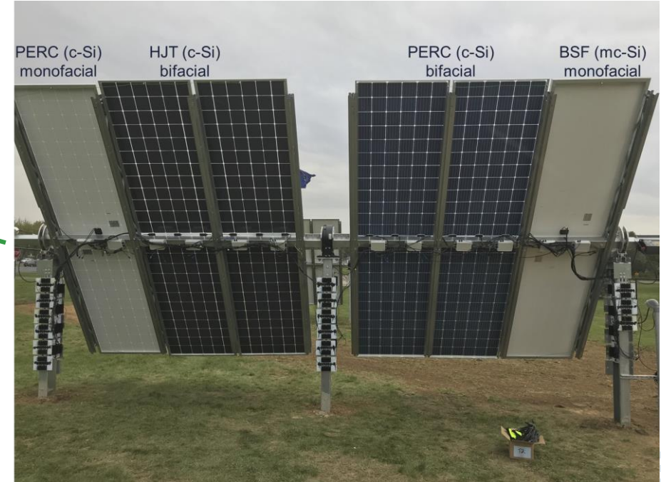
Modules under test
