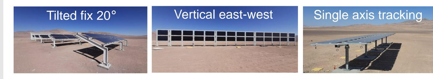
MW PV Plant with HSAT. **25%** of possible change in the plant for R&D investigation
