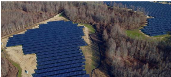
Sunpreme PV Power Plant (commercial), USA 3
