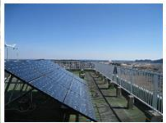
Thin film Si PV 4 kW KANEKA Corporation
