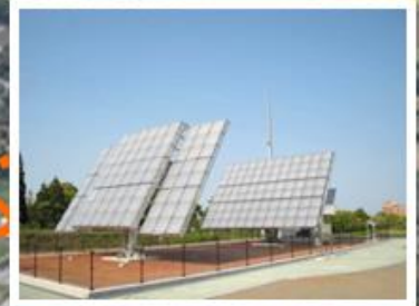
CPV 10 kW × 2 systems Sumitomo Electric Industries, Ltd.
