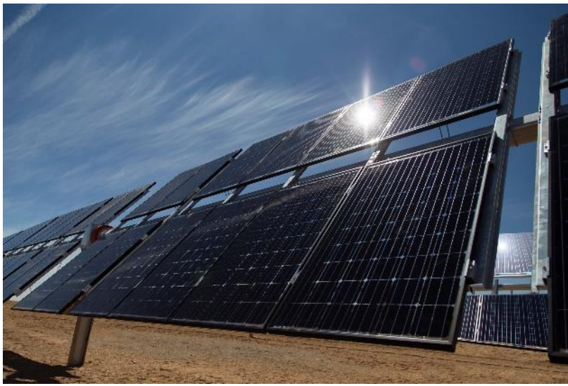
'La Silla' solar plant (Chile), 2015. Soltec produced the first solar tracker specifically designed for bifacial modules installed in a utility scale solar plant.
