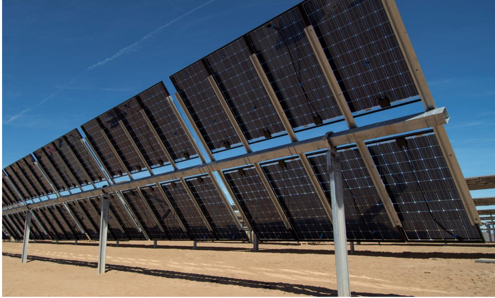
'La Silla' solar plant (Chile), 2015. Soltec produced the first solar tracker specifically designed for bifacial modules installed in a utility scale solar plant.
